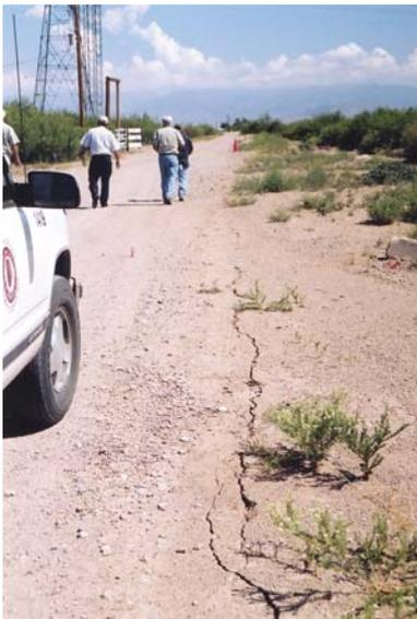
**Figure 1.** Initial crack that formed along Nickels Road north of Willcox. View is to the north with Mount Graham in the background. Normally dry wash is on the right side of the road. Photograph was taken July 20, 2004.
