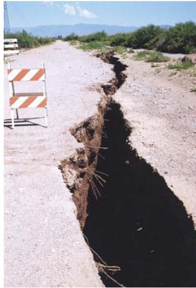
**Figure 2.** The desiccation crack shown in Figure 1 was enlarged when runoff from the wash flowed into it. Photograph taken from the same spot as in Figure 1, only a few days later.
