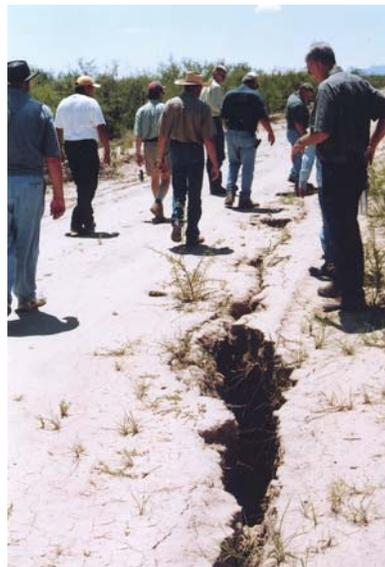
**Figure 4.** A large desiccation crack has developed along a private road south of Dragoon Road west of U.S. Highway 191. This crack has been present for several years.
