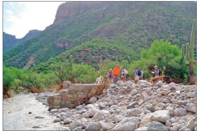
**Figure 6.** A large debris flow that came down Rattlesnake Canyon into Sabino Creek completely blocked the Rattlesnake Creek Bridge with coarse sediment and eroded the northern approach of the tram road. The people are standing on the bridge; Sabino Creek is behind them.
